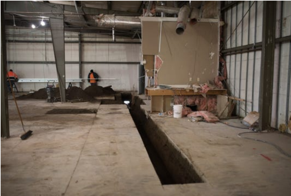
Construction workers begin work on the Family Resource and Child Development Center in Salem. The center, which will serve as a hub of resources for local families, will be located at the corner of Portland Road NE and Bill Frey Drive in the old old St. Vincent de Paul building. (Photo: Courtesy of Nathan Schwab, Catholic Community Services)
