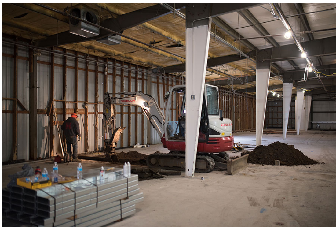
Workers get going on a project to renovate a former Salem St. Vincent de Paul building into a family resource and child development center to be operated by Catholic Community Services in Salem. (Courtesy Catholic Community Services)
