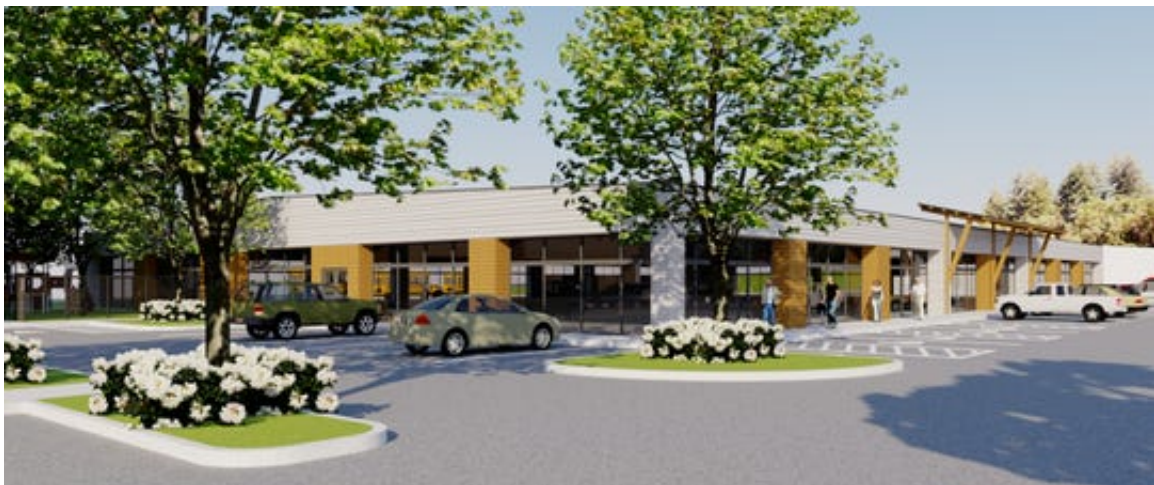
A rendering of the future Family Resource and Child Development Center, run by Catholic Community Services, that will be located off Portland Road NE in Salem. The center is expected to have a partial opening in August, 2019, with a full opening in January, 2020. (Photo: Courtesy of architect Ron Ped)
