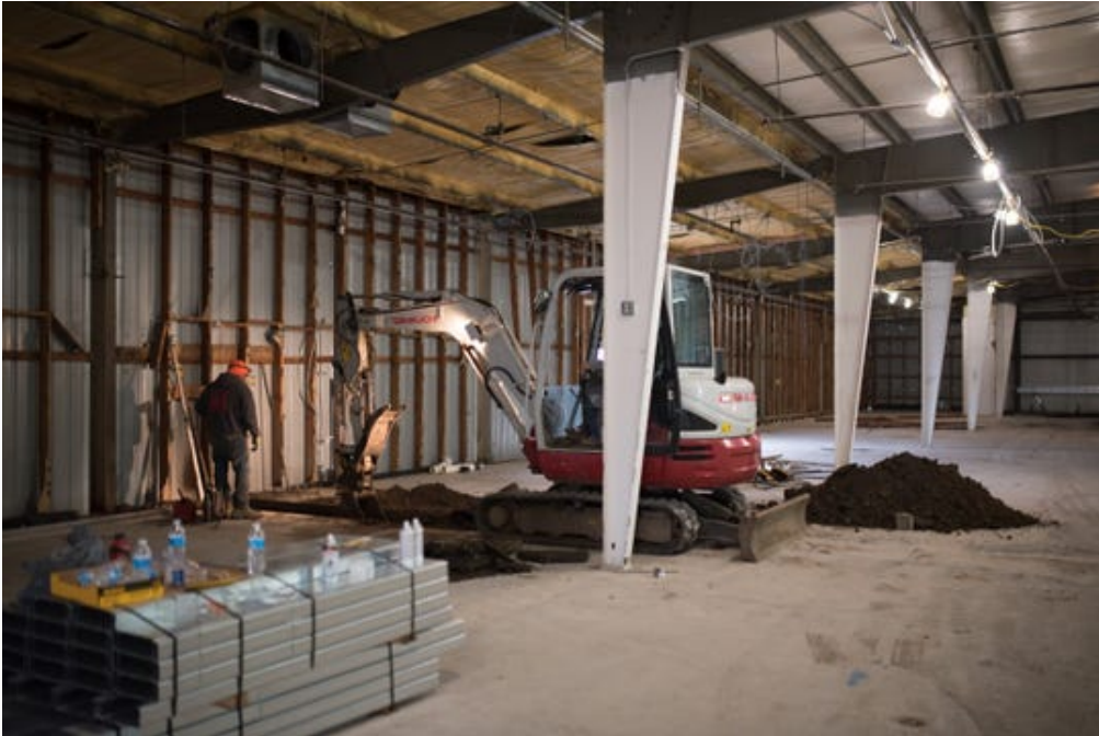
Construction workers begin work on the Family Resource and Child Development Center in Salem. The center, which will serve as a hub of resources for local families, will be located at the corner of Portland Road NE and Bill Frey Drive in the old St. Vincent de Paul building. (Photo: Courtesy of Nathan Schwab, Catholic Community Services)
